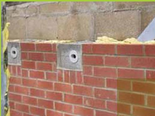
Schwegler Swift Bricks installed in sheltered housing in London
