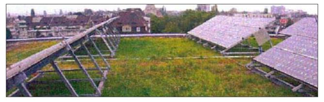
However, the use of a Green Roof maintains the ambient temperature at roof at about 25°C allowing the PVs to work at optimum efficiency
