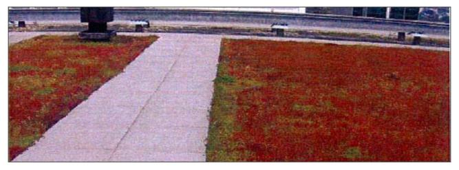
The roof was partially planted with a sedum mat to provide resistance to soil erosion due to the wind on the exposed site. The use of the wildflower mix in the substrate meant that as the roof matured a wide range of plants developed avoiding the monoculture of sedum mats.
