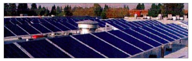
Gregg et al. while researching PV efficiencies for United Solar Ovonic LLC, found the performance of photovoltaic panels is lowered by 0.5%/°C above or below 25°C. Therefore at 600°C the efficiency is reduced by 17.5% affecting the payback period and economic viability of PVs.
