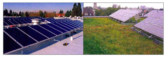
If we bring these two pictures together, it's fairly obvious how hot the uncovered roof can be and it is easy to appreciate how a Green Roof conditions the air and improves the efficiency of solar energy collection panels.
